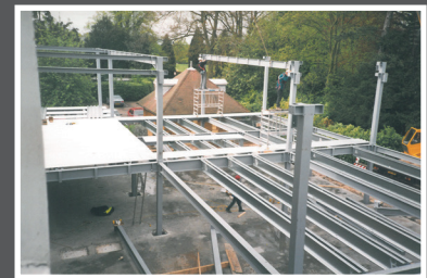
Construction of the Sherbourne
